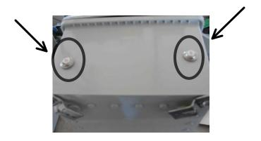
Outside, on the bottom, are 2 more circuit breakers. If either of these trip, no motors will run. If tripped, reset by pressing the operator in.
